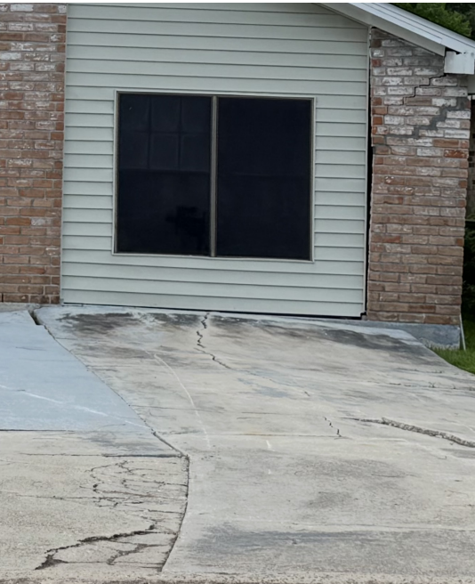
Figure 19. Home with damaged foundation resulting from flooding and subsidence. Photo Credit: St. Mary Excel
